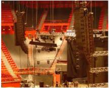
Figure 74: Hybrid flown/stacked subwoofer example: L/R = 14 V-DOSC + 3 dV-DOSC (per side); flown dV-SUB (6 per side); ground stacked SB218 (6 per side); LL/RR = 4 V-DOSC + 6 dV-DOSC (per side); stereo infill = 2 dV-DOSC (per side); distributed front fill = 4 dV-DOSC (Bjork, POPB Paris 2003 – sound design M Malki)
